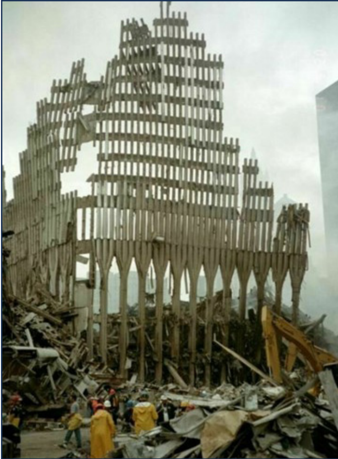
Figure 2: The "Fence." The remaining structural facade of Tower 2.
