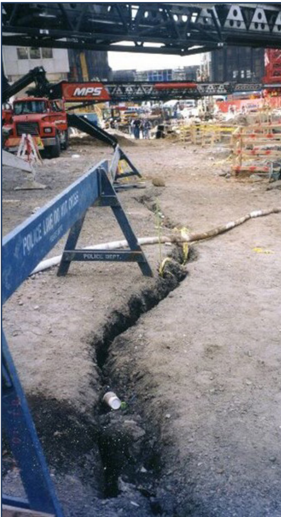
Figure 8: The appearance of a fissure in the street signaled movement of the slurry wall and triggered an immediate response to stabilize it.
