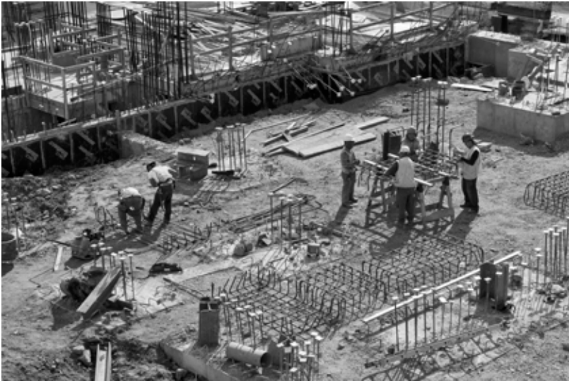
LEFT Rebar being laid out at the WTC site.
